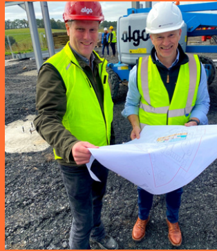
Chris Stewart (Chris Stewart Group) and Andrew Bateman (3DReid) checking plans on site.
